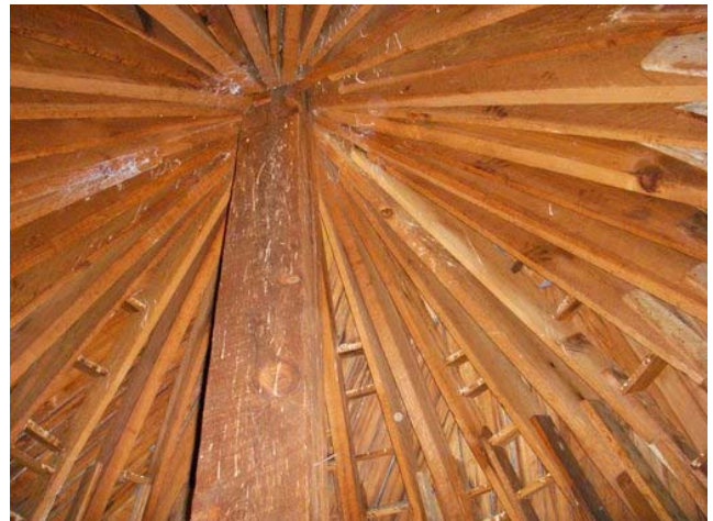
Heart Pine Beam and Joists Supporting the Clock Tower Dome
