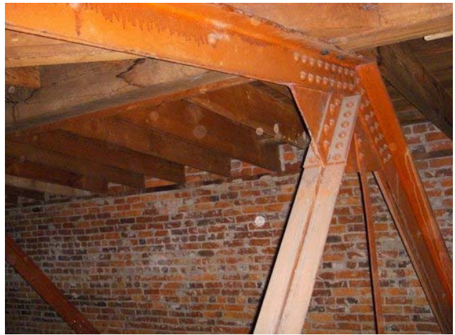
Steel Struts Supporting Heart Pine Beams in Belfry
