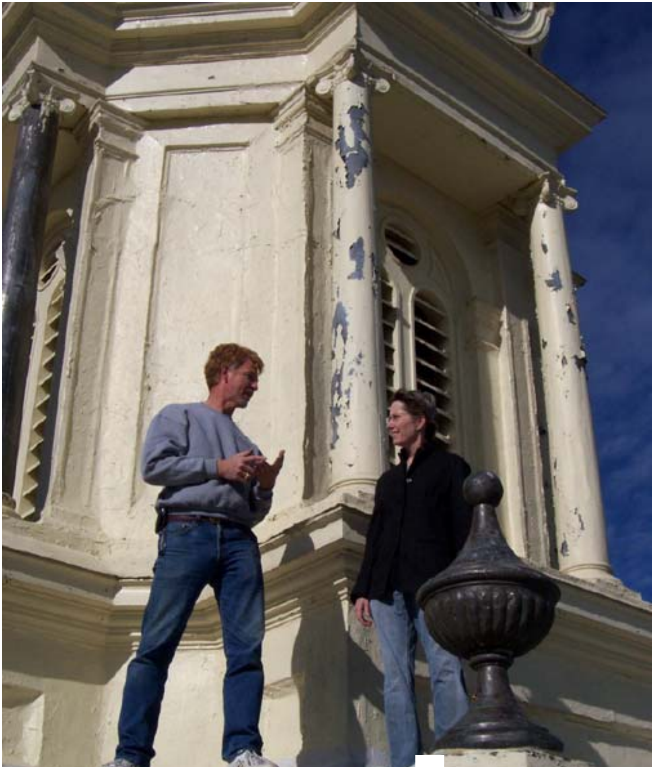
Burles Johnson explains restoration techniques to Helen Aikman during tour of the Courthouse clock tower restoration. Photo by Robert Yonchak.
