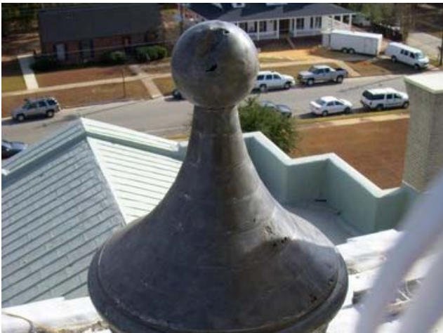
Stripped Finial with Partly Restored Standing Seam Roof in Background
