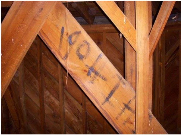
Heart Pine Beam Scrawled with Courthouse Construction Date
