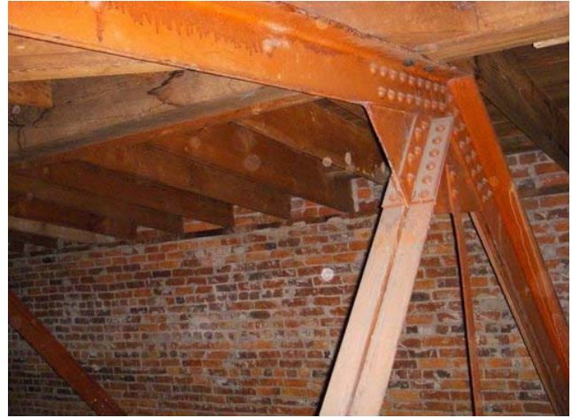
STEEL STRUTS AND HEART PINE BEAMS IN BELFRY
